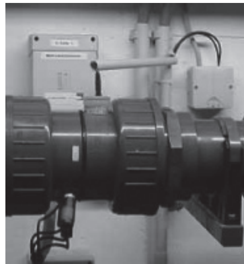
Fig. 6-2: Arranging the electrolysis cell after it has been installed
